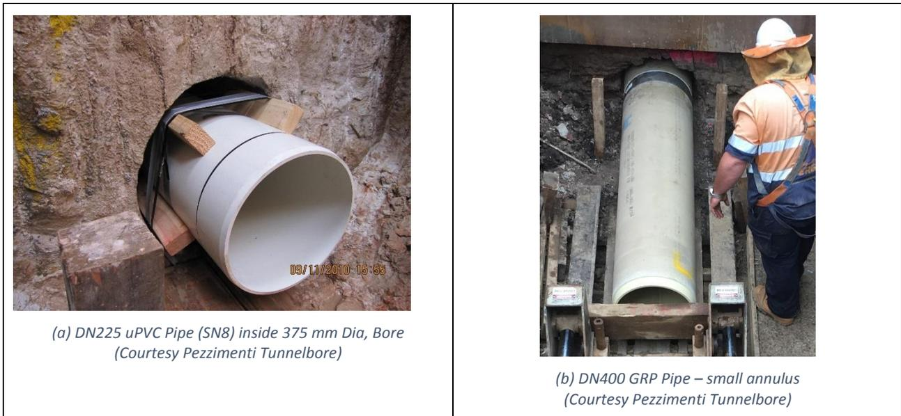
Figure 5 - Examples of Slip Lined Pipes Inserted into Excavated Bores
