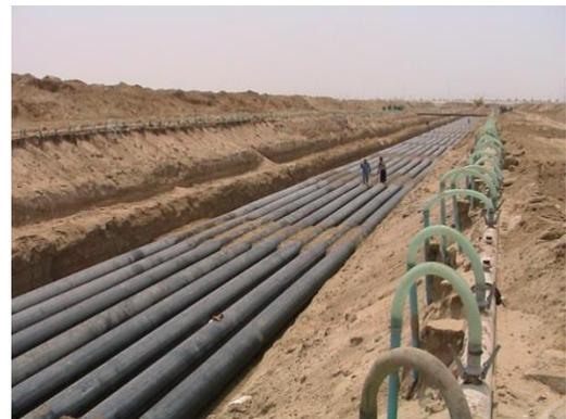
As there are no 1200mm pipe extruder available during that time 4 parallel line of 630mm were designed in place to one 1200 ID GRP pipes. The new design was fit for the purpose and also provided flexibility to the operator to use individual lines depending on the load.
